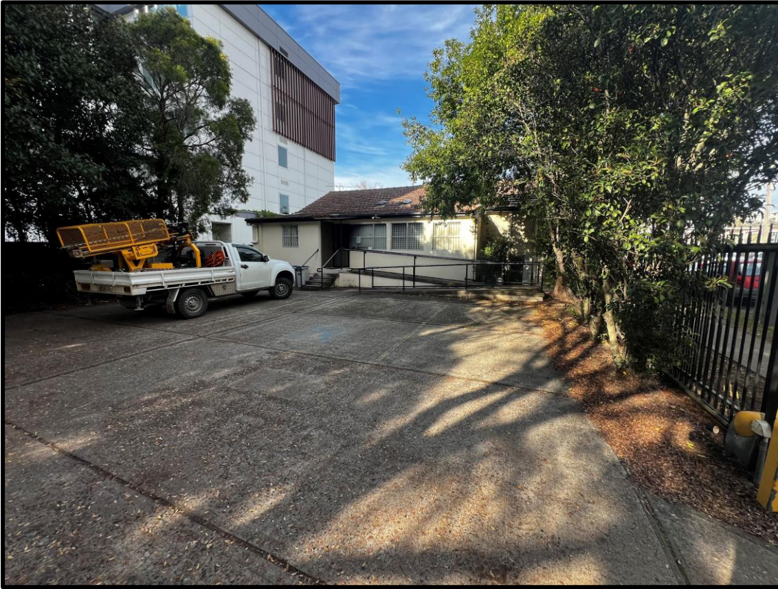
Figure 10. Parking with concrete groundcover within the rear of the site.
