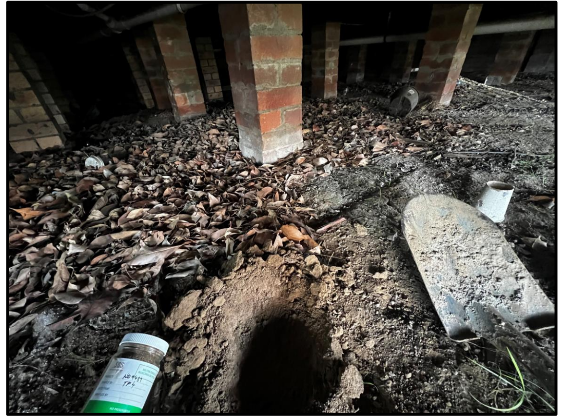
Figure 13. Test pit excavation of TP4 underneath onsite building
